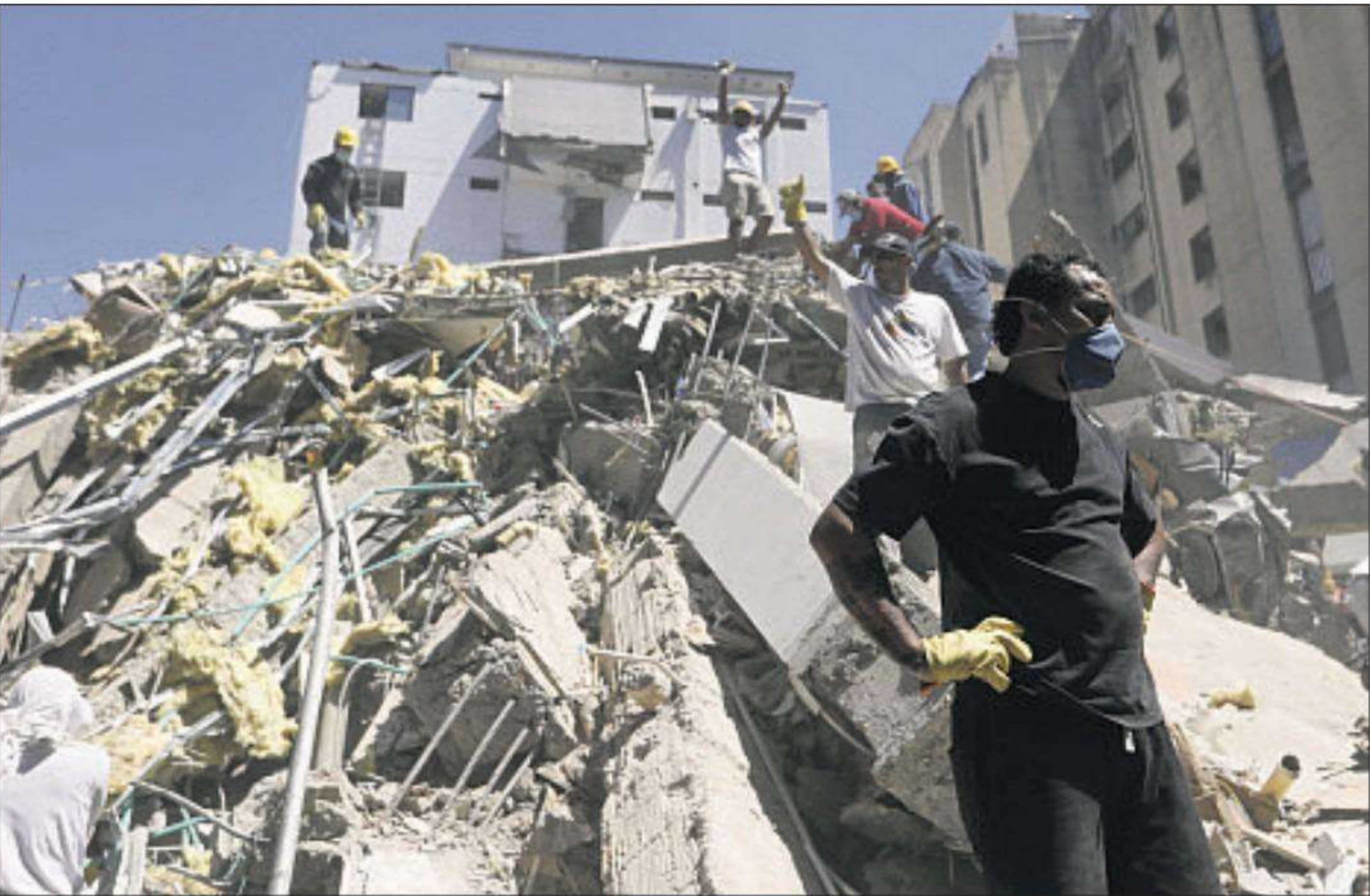
RESIDENTS and rescue workers search through the rubble after an earthquake struck Cali, Colombia.
